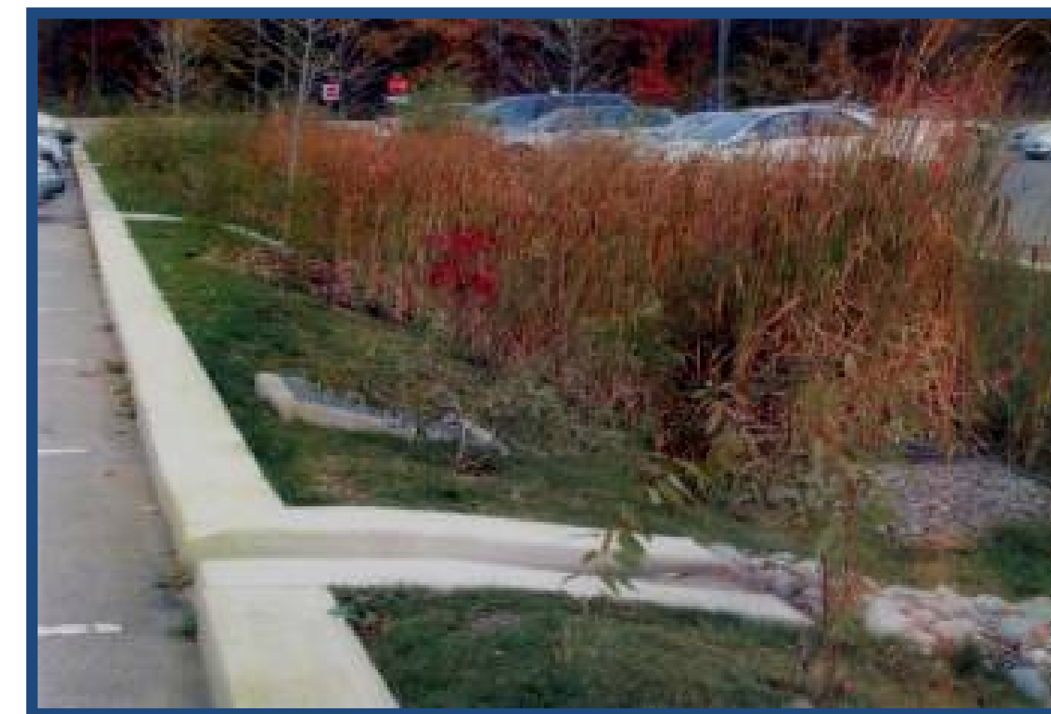
Bio-retention Facility To Treat Parking Area
