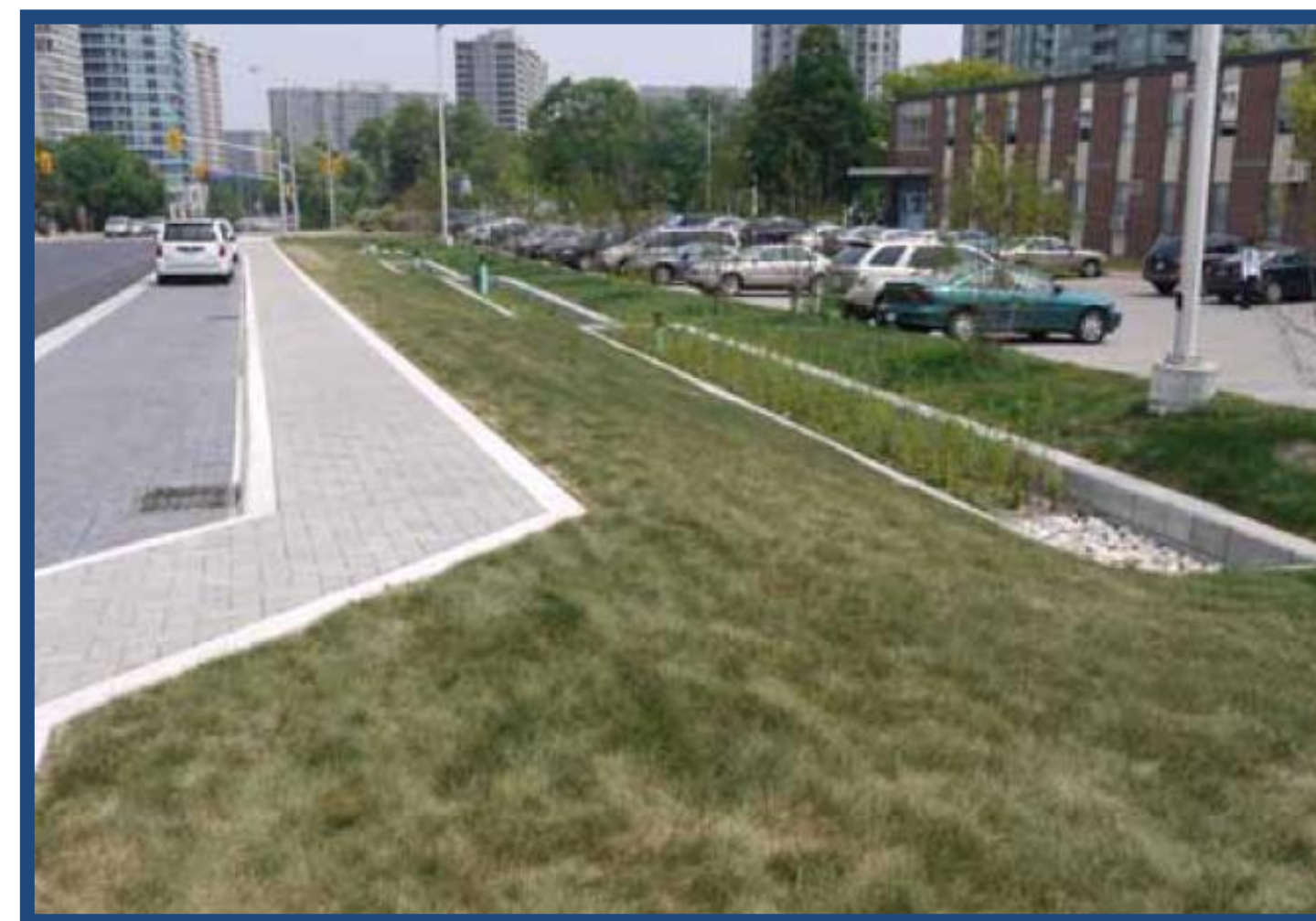
Bio-retention Facility To Treat Roadway Drainage
