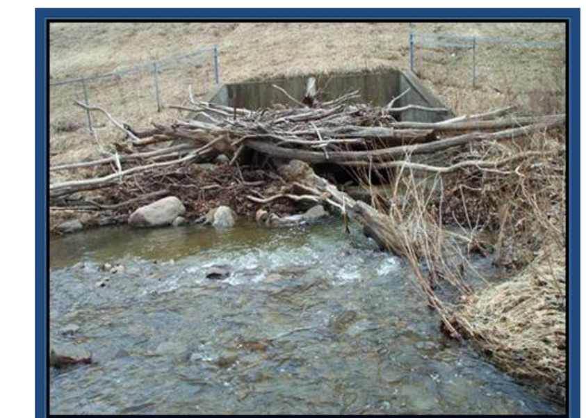
Culvert Blocked with Debris
