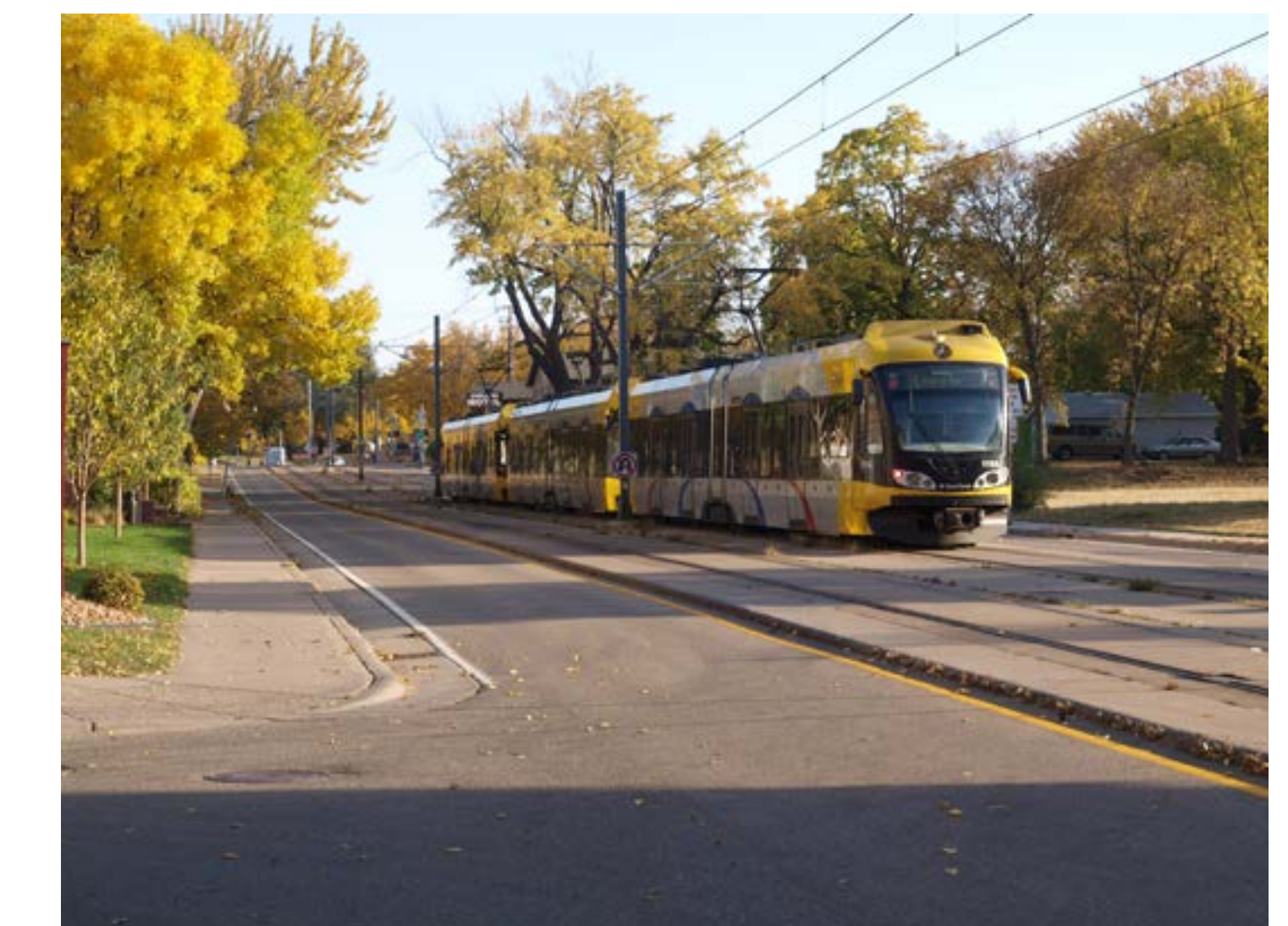
Centre-pole catenary system in Minneapolis (centre-running with one traffic lanes on each side)
