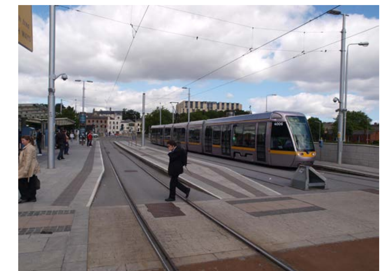
Side-pole system at off-street stop in Dublin with platform lighting combined on OCS poles
