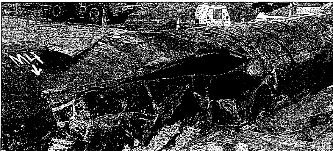
Above: The ruptured section of Enbridge's failed pipeline in Michigan, excavated following the July 2010 spill.
